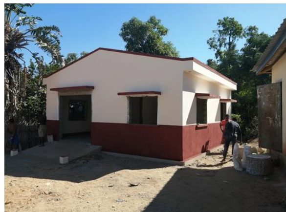
Wharehouse construction completed
