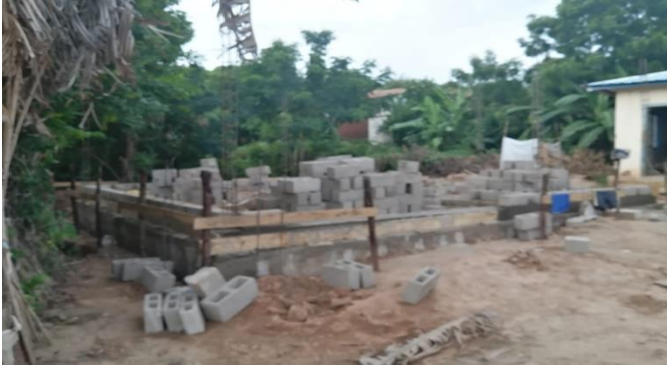
Warehouse initial construction
